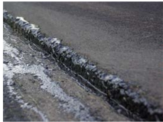
Figure 11. Joint adhesive application on milled joint.
