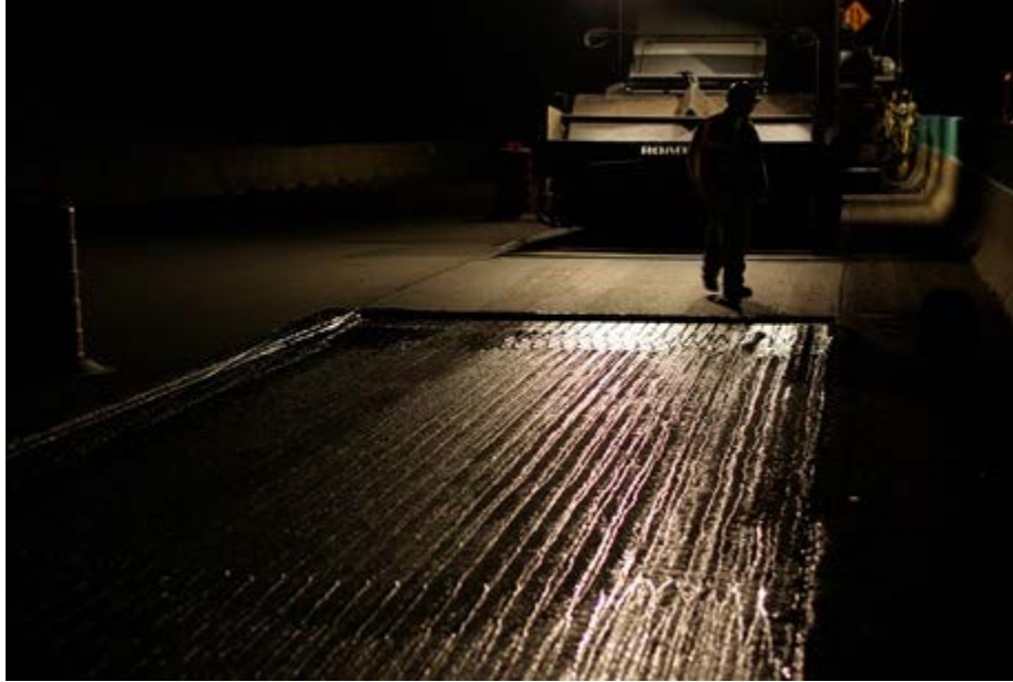
Figure 7. Straight PG grade tack coat placement.
