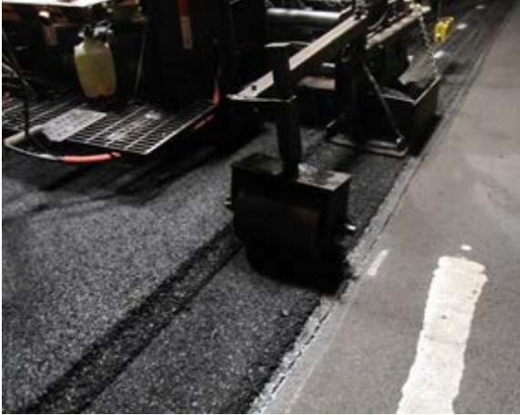
Figure 8. Notched wedge joint.
