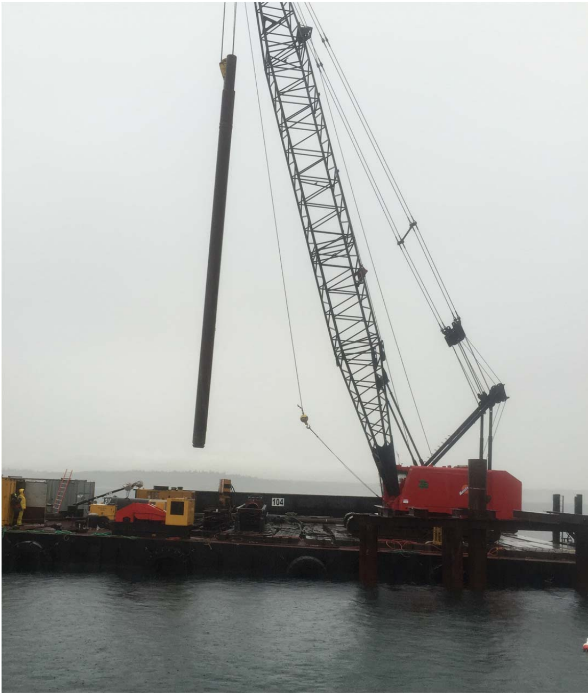
Figure 5: Crane lofting double-walled pile into place. Photo courtesy Jim Laughlin, WSDOT.
