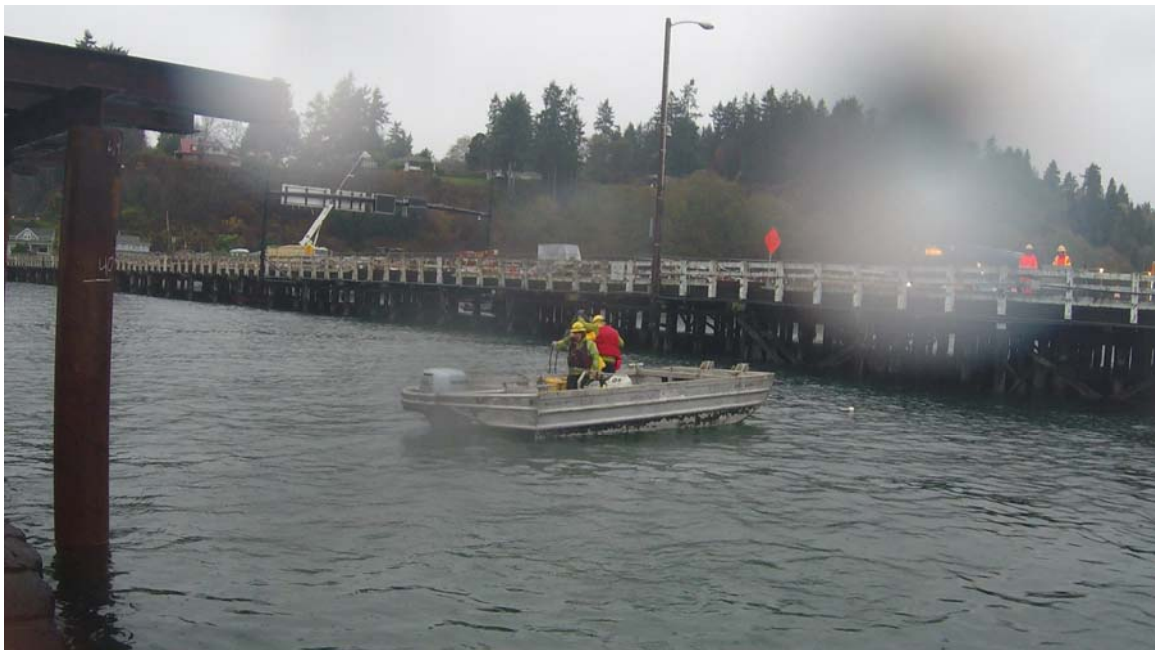
Testing at Vashon Island Ferry Terminal
