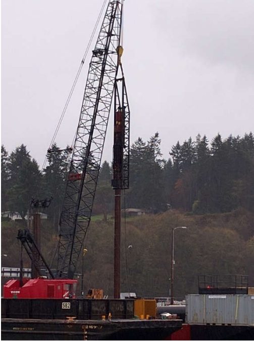
Figure 3a. The placement of the impact hammer on the control pile, taken from the R/V Robertson on 7 December.
