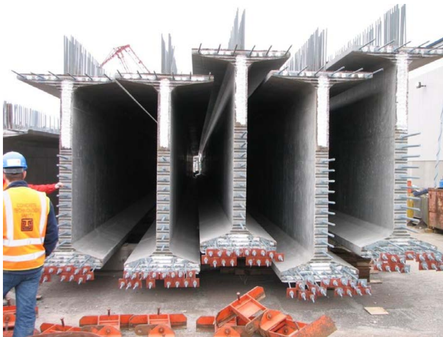
Figure 1.1: Extended Girder Strands for Positive Longitudinal Seismic Moment Connection in Washington State
