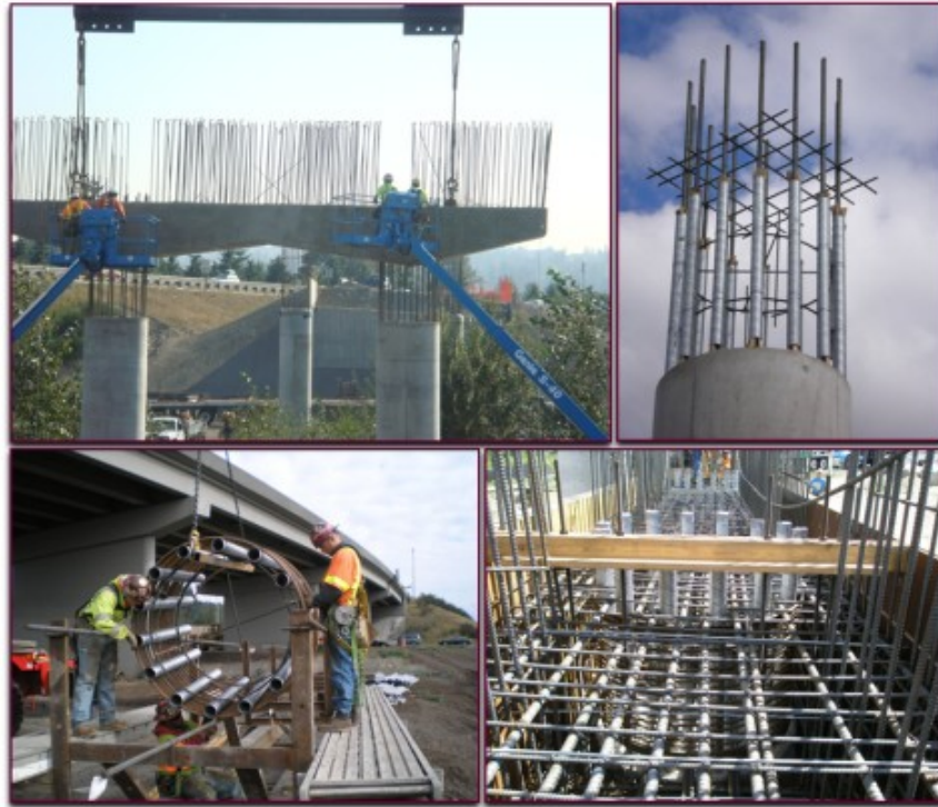
Figure 1.2: Precast Bent Cap Construction in the State of Washington
