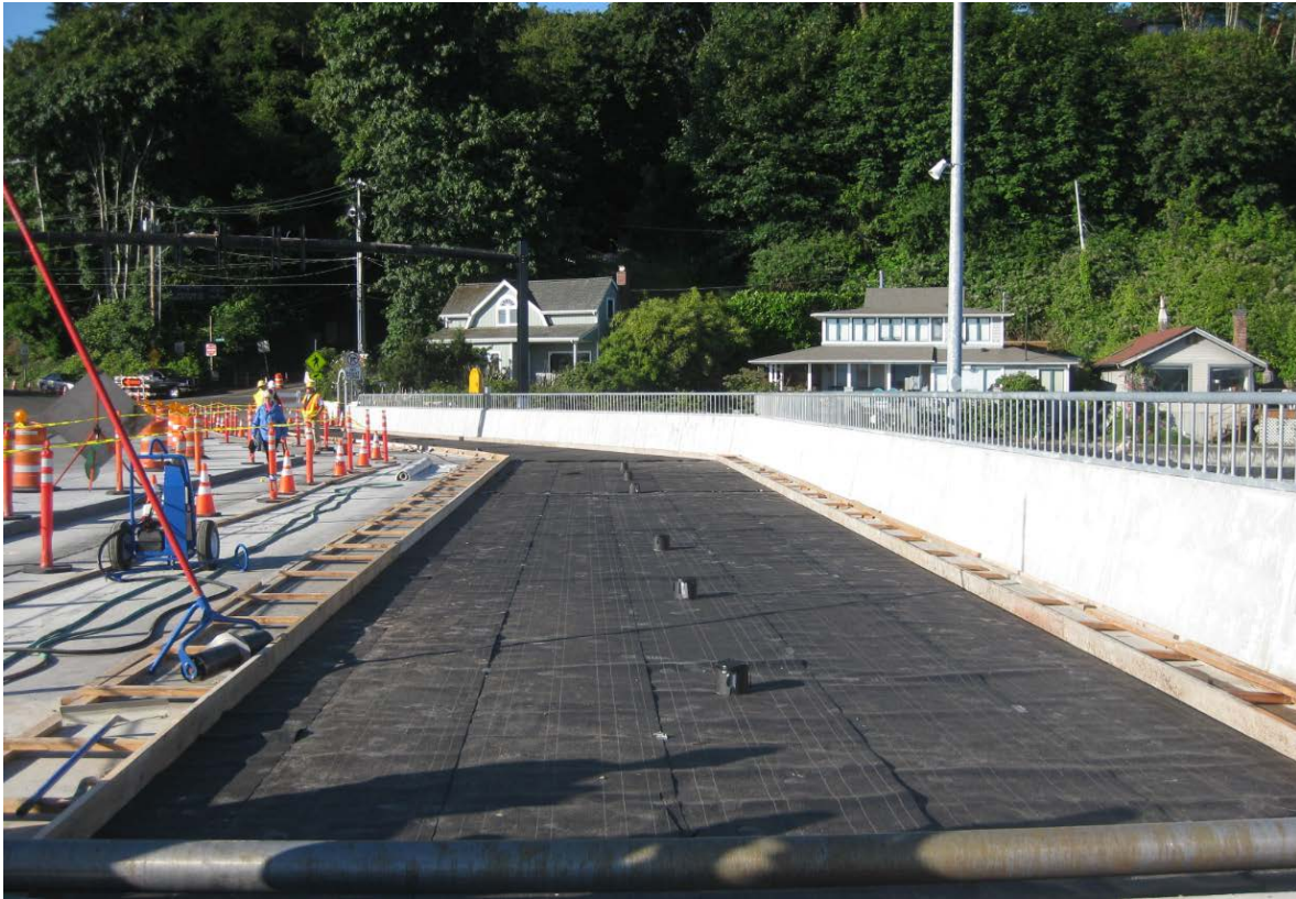
Figure 6- Southbound lane under construction on June 17 2016.
