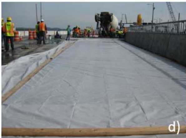
Figure 7- (a) Finishing PC flat using a vibratory roller. (b) Roller compacting PC. (c) Joints cutting. (d) Freshly placed PCP covered with plastic sheets for curing. (e) Hardened PCP in the outer lane after the curing period.
