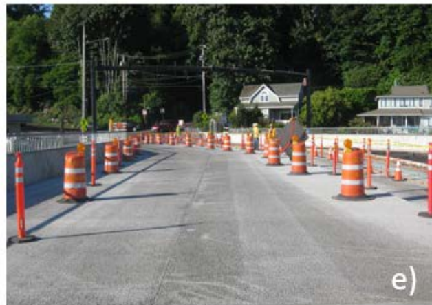
Figure 7- (a) Finishing PC flat using a vibratory roller. (b) Roller compacting PC. (c) Joints cutting. (d) Freshly placed PCP covered with plastic sheets for curing. (e) Hardened PCP in the outer lane after the curing period.
