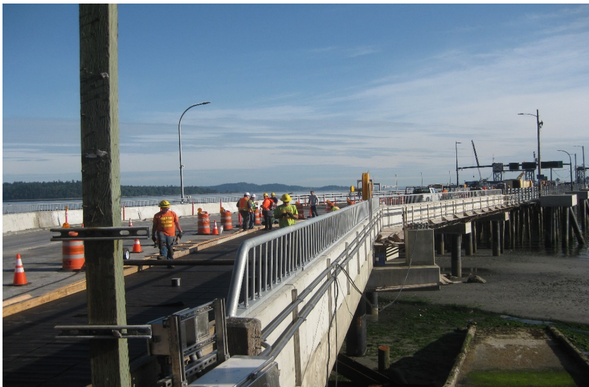
Figure 5- Northbound lanes under construction on June 1 2016.
