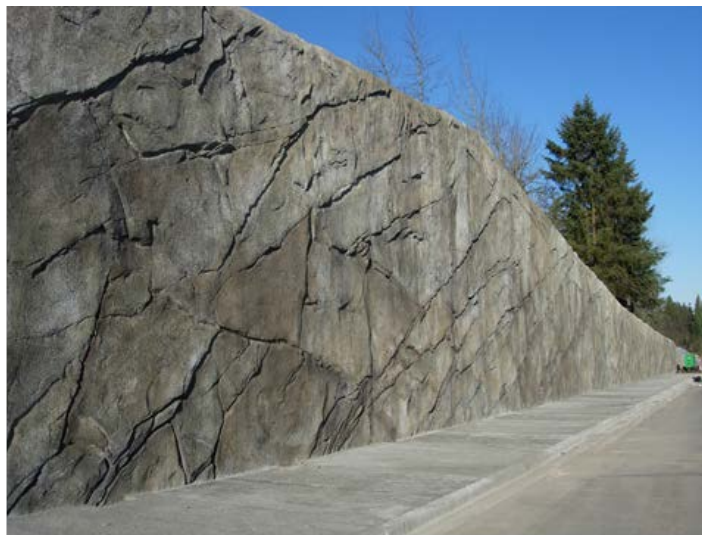
Figure 1.1 Shotcrete retaining fascia walls
