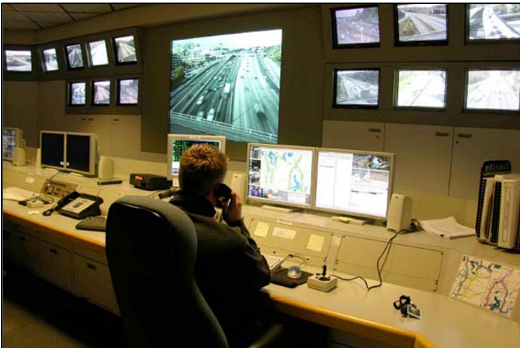
Figure 1: WSDOT Traffic Management Center
