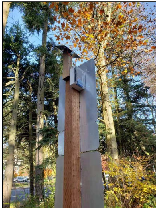
Figure 5.3: Smart Road Sticker in its case and a solar panel mounted on the southwest side of the trail
