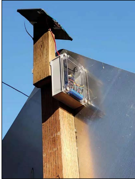
Figure 5.2: Smart Road Sticker in its case and a solar panel mounted on the northeast side of the trail
