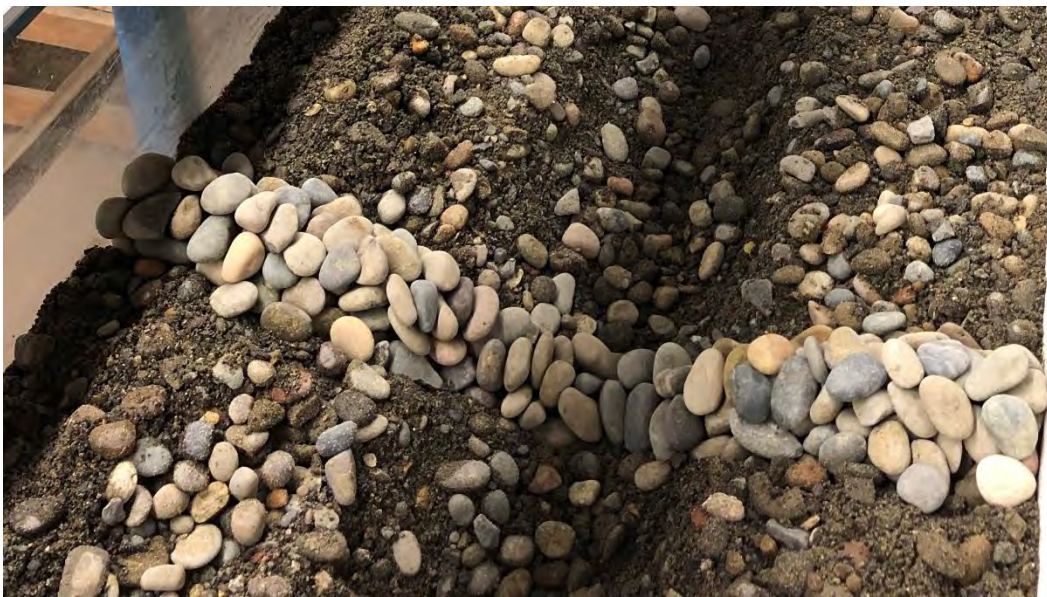
Figure 7 Coarse band design that replicates the channel shape and sits about the streambed 1.5-2 particle diameters.
