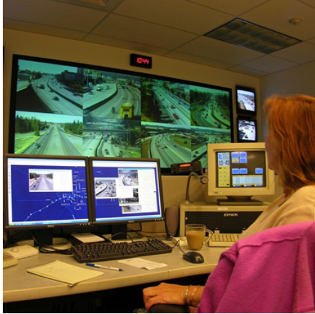
Monitoring highway traffic and safety conditions.
