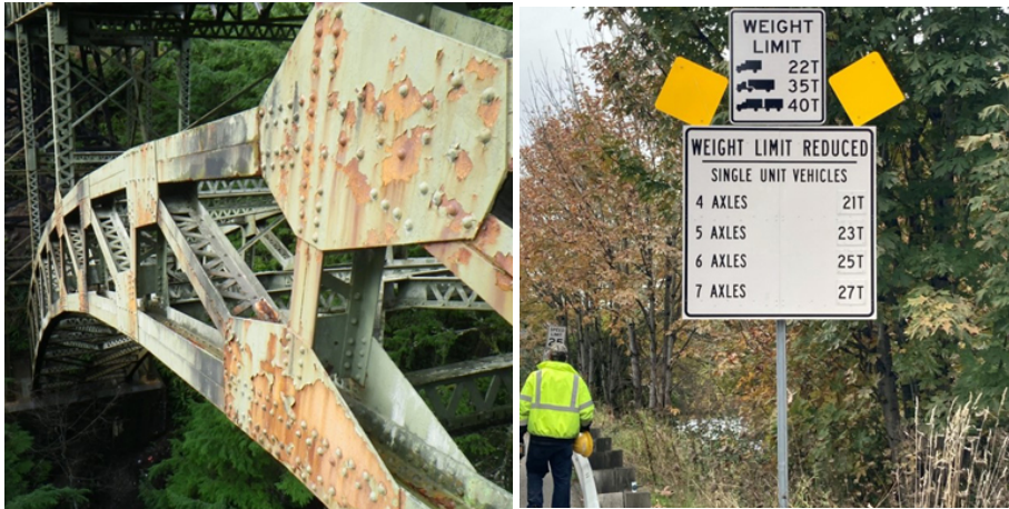
Examples of a load posted bridge.
