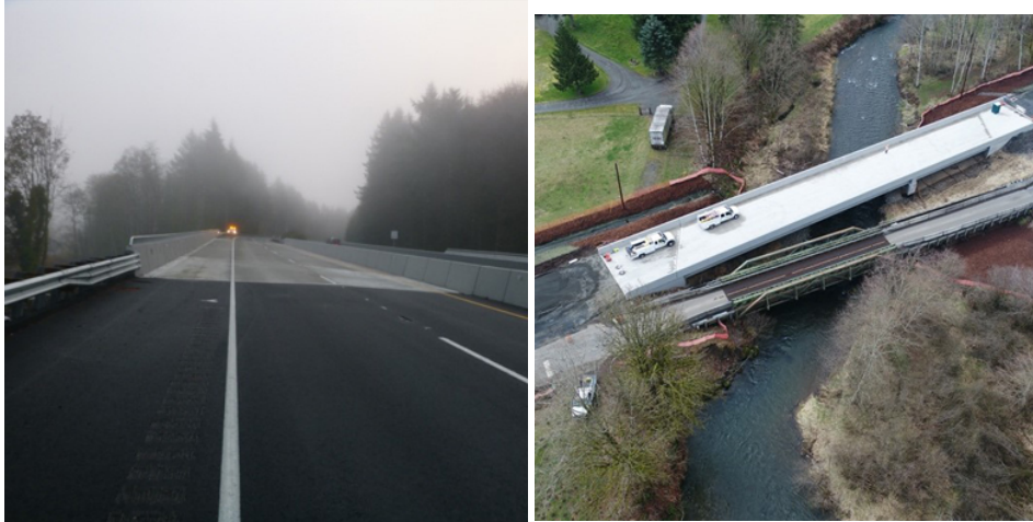
Examples of well-funded bridges in good condition.
