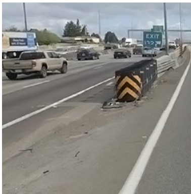
Example of well-maintained highway crash cushion.
