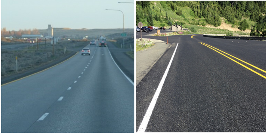
Examples of pavement in good state of repair.
