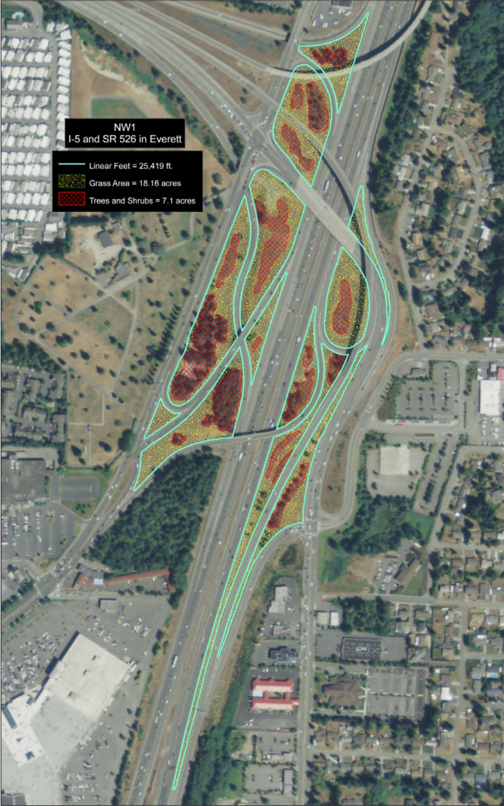
Figure 3. NW1: I-5 @ SR 526 Interchange
