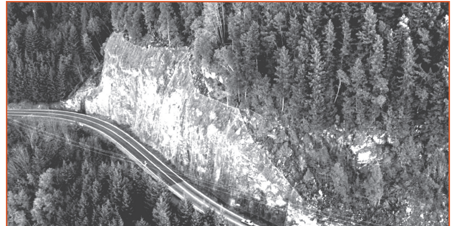
A study developed guidelines for using draped wiremesh and cablemesh slope protection systems, such as this mesh system north of Vancouver, B.C., installed to direct falling rock into an accumulation ditch.
