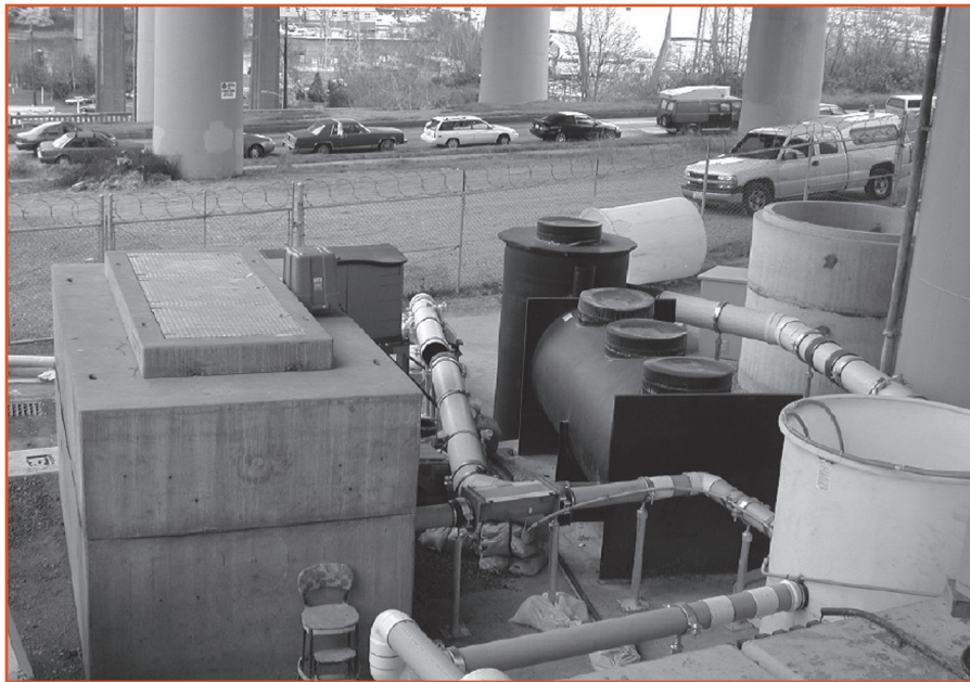
An innovative research facility located below the Ship Canal Bridge in Seattle is testing the quality of highway water runoff subjected to different stormwater treatments.
