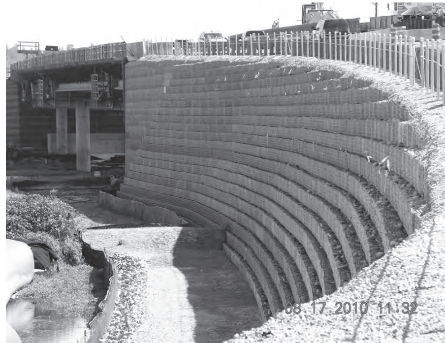
Completed retaining wall for a new bridge on SR 532 in western Washington. (Photo by WSDOT)
