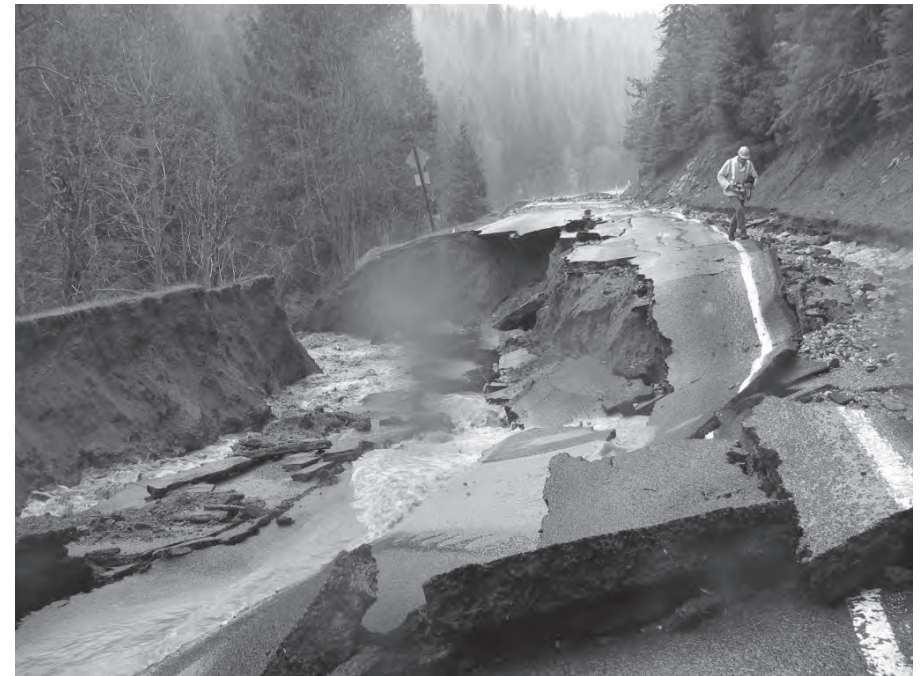
Workers inspect a washout on SR 206. Researchers are developing a baseline assessment of climate change impacts on transportation condition and serviceability in the Pacific Northwest and Alaska. (Photo by WSDOT)
