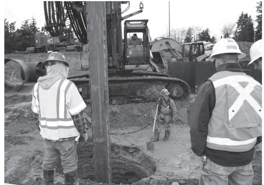
Crews drill a shaft for a bridge column in Tacoma, Washington. (Photo by WSDOT)
