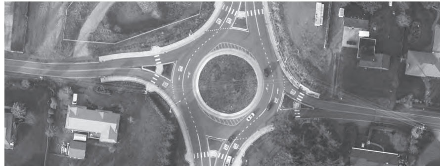
SR 539, Wiser Lake Road Roundabout near Lynden, Washington. (Photo by WSDOT)
