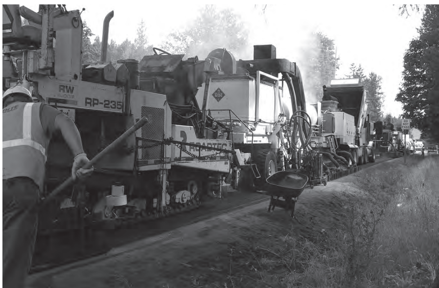
Hot in-place recycling successfully rehabilitated the pavement on SR 542 while using less new material than the traditional hot mix asphalt process. (Photo by WSDOT)
