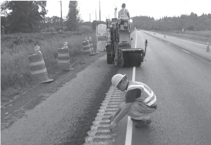
Centerline rumble strips (here being placed on a shoulder of US 2) were found to be an effective, low-cost, low-maintenance countermeasure that reduces the frequency of collisions. (Photo by WSDOT)
