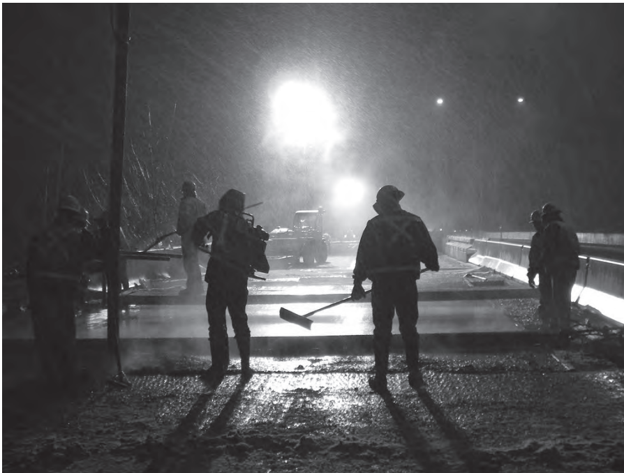
On busy SR 520 in Seattle, pavement repair that closes the freeway must occur at night. Researchers are upgrading the CA4PRS software, designed to help engineers better design, analyze, and construct long-lived pavements while minimizing traffic delays. (Photo by WSDOT)
