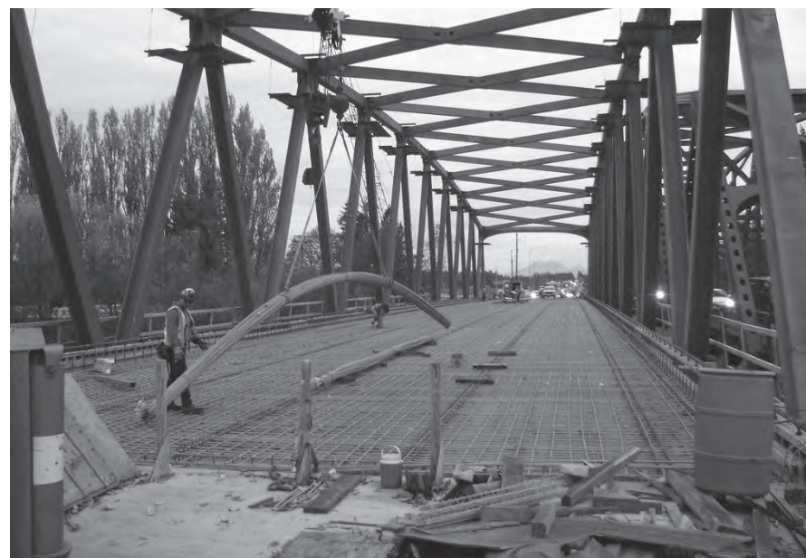
Crews install steel rebar on a bridge in Washington. Deicers may corrode rebar. Research concluded that the best prevention may be less permeable concrete, rather than more expensive, corrosion-inhibiting deicers. (Photo by WSDOT)
