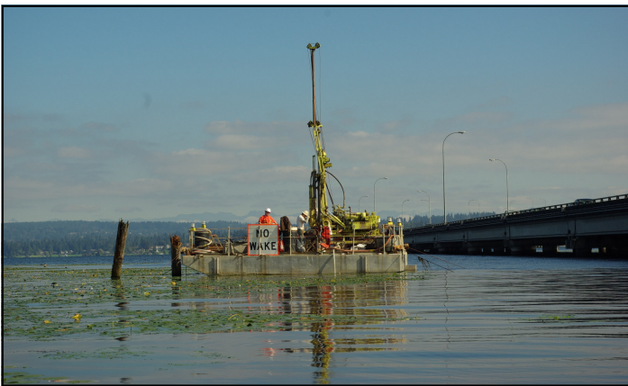
Crews will use barge-mounted geotechnical equipment.
