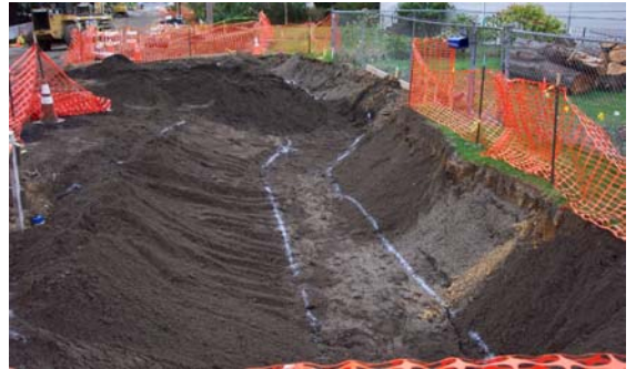
Grading – 2-foot shoulder then 3H:1V road side
