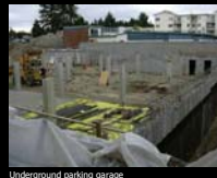
Underground parking garage
