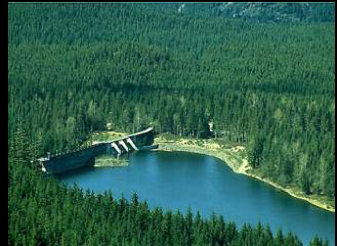
The Cedar River Reservoir
