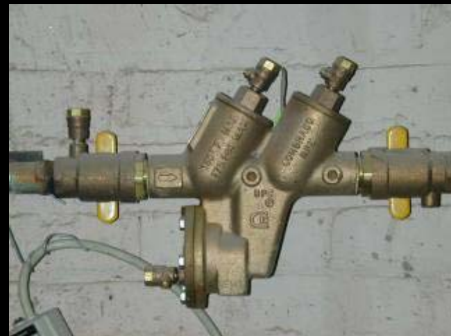
Reduced pressure principle backflow assembly
