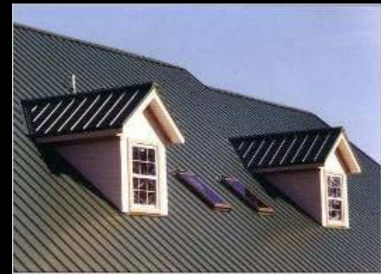
Standing seam metal roof
