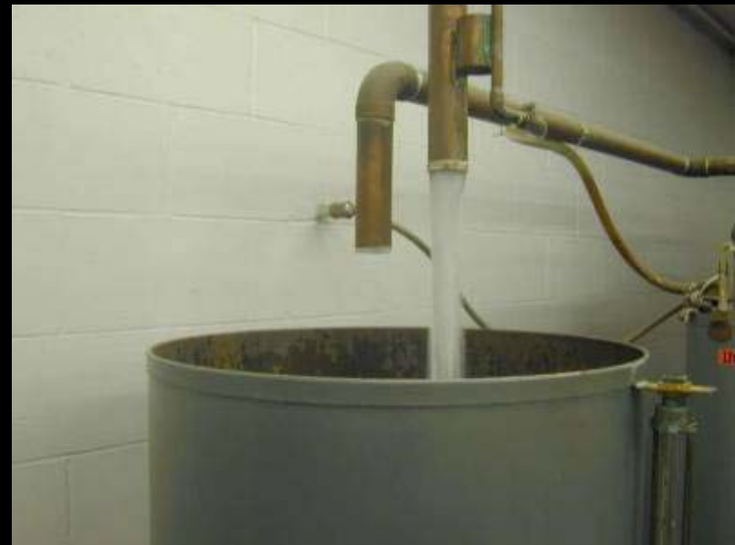
An air gap between rainwater cistern and potable back-up
