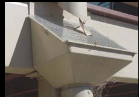
Self cleaning course pre-treatment screen
