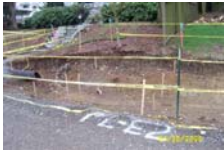
Swale subgrade excavation
