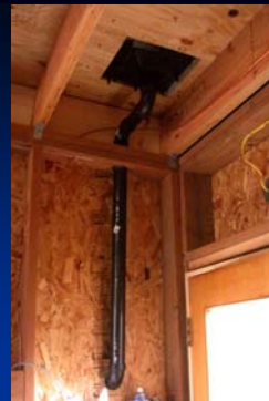
Roof Drain - Interior
