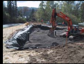
Large Raingarden for handling street run-off
