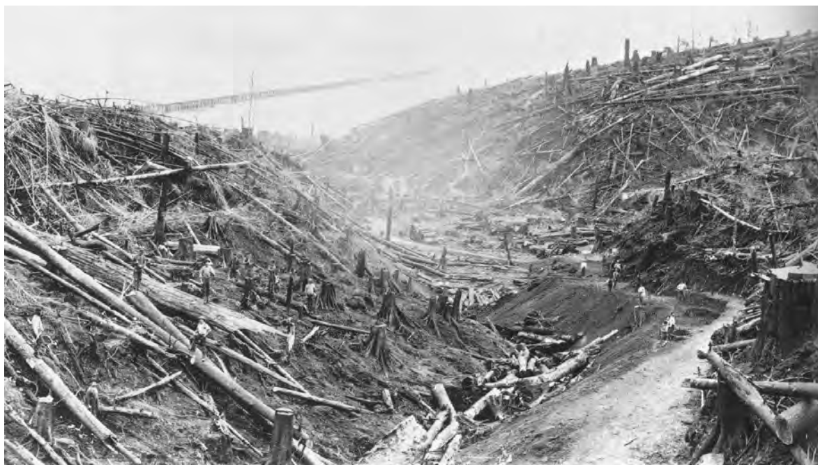
Figure 3-13. View of Grays Harbor City wharf on 19 August 1889 from of a ravine logged in anticipation of the establishment of a boom town serving rail and sea-going traffic. Wharf extends 1 mile to a deep-water channel. (University of Washington Libraries, Special Collections, Order Number WAS1276, Negative Number UW4363)
