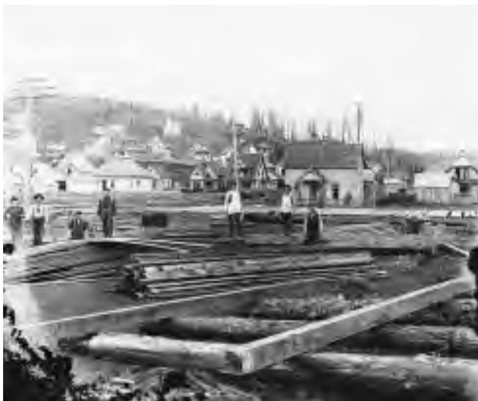
Figure 3-11. Construction of streets in Hoquiam c. 1908, using planking necessary to keep them out of reach of high tides. (University of Washington Libraries, Special Collections, Order Number WAS0195, Negative Number UW348)
