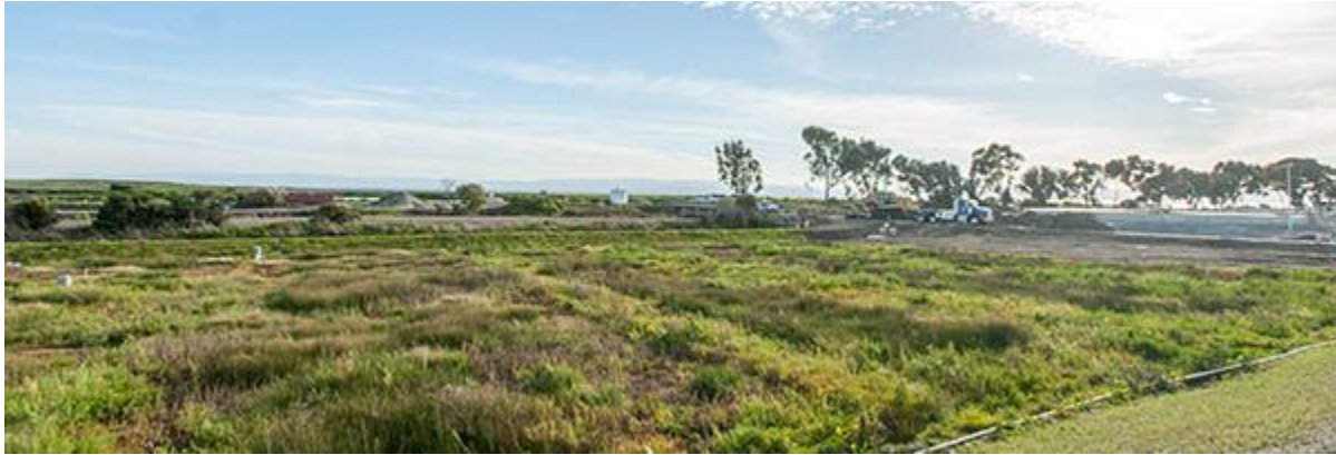
Figure 31: Oro Loma Horizontal Levee Project in San Lorenzo, CA, where restoration of native vegetation is utilized for treating incoming wastewater at a local sanitary district. Source: https://oroloma.org/horizontal-levee-is-thriving/
