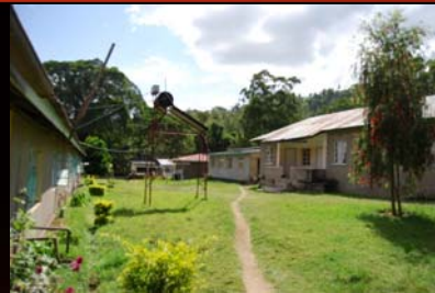
Courtyard between the ward and cafeteria
