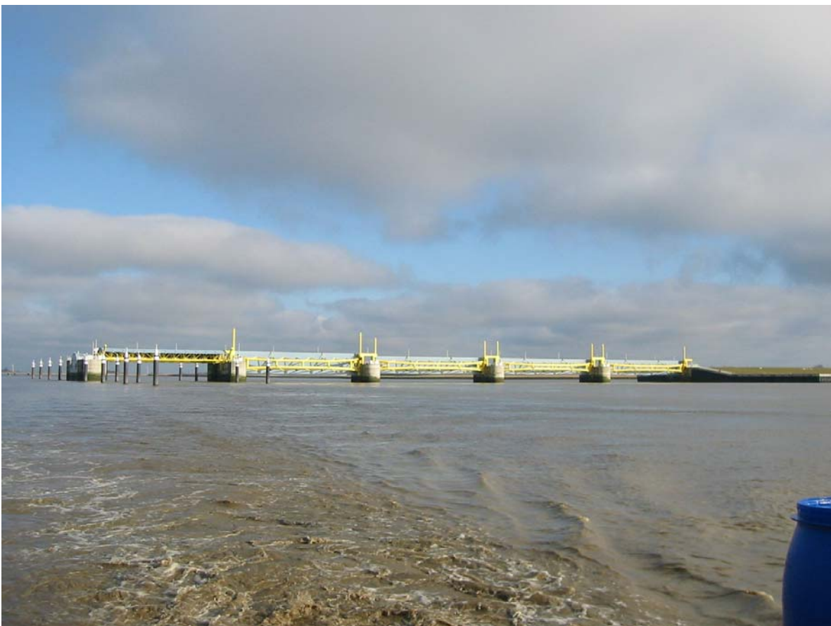
Figure 3.5. Photograph of the Emssperwerk in March, 2005. Note the turbid water in the foreground.
