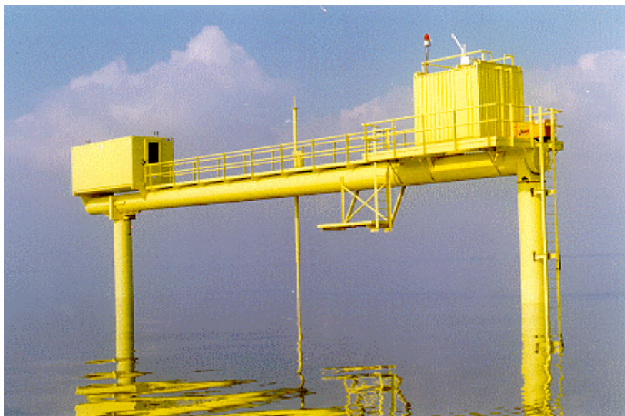
Figure 4.1 Picture of the BOA bridge
