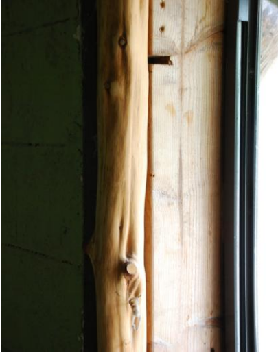
Figure 14. Aliz finished cobb walls
