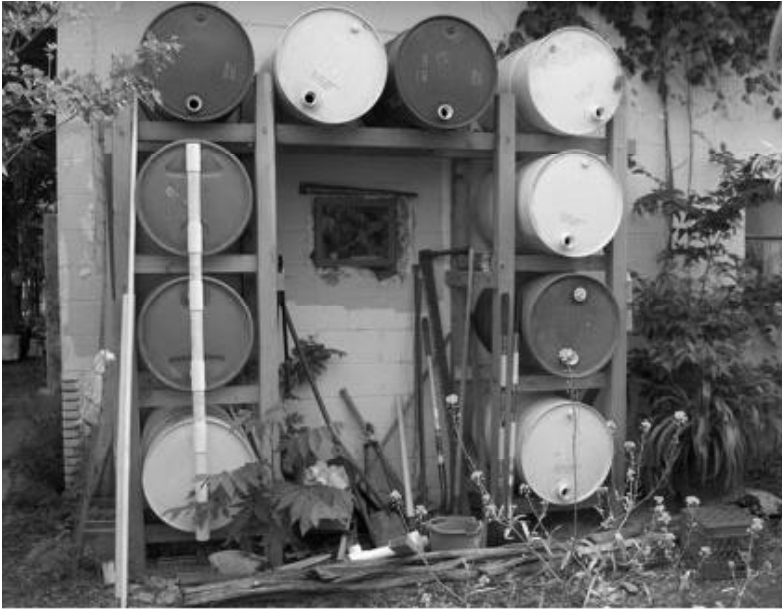
Figure 9. Harvested Water Storage Structure 48
