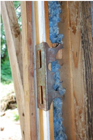
Figure 17. Construction of cobb wall 50
