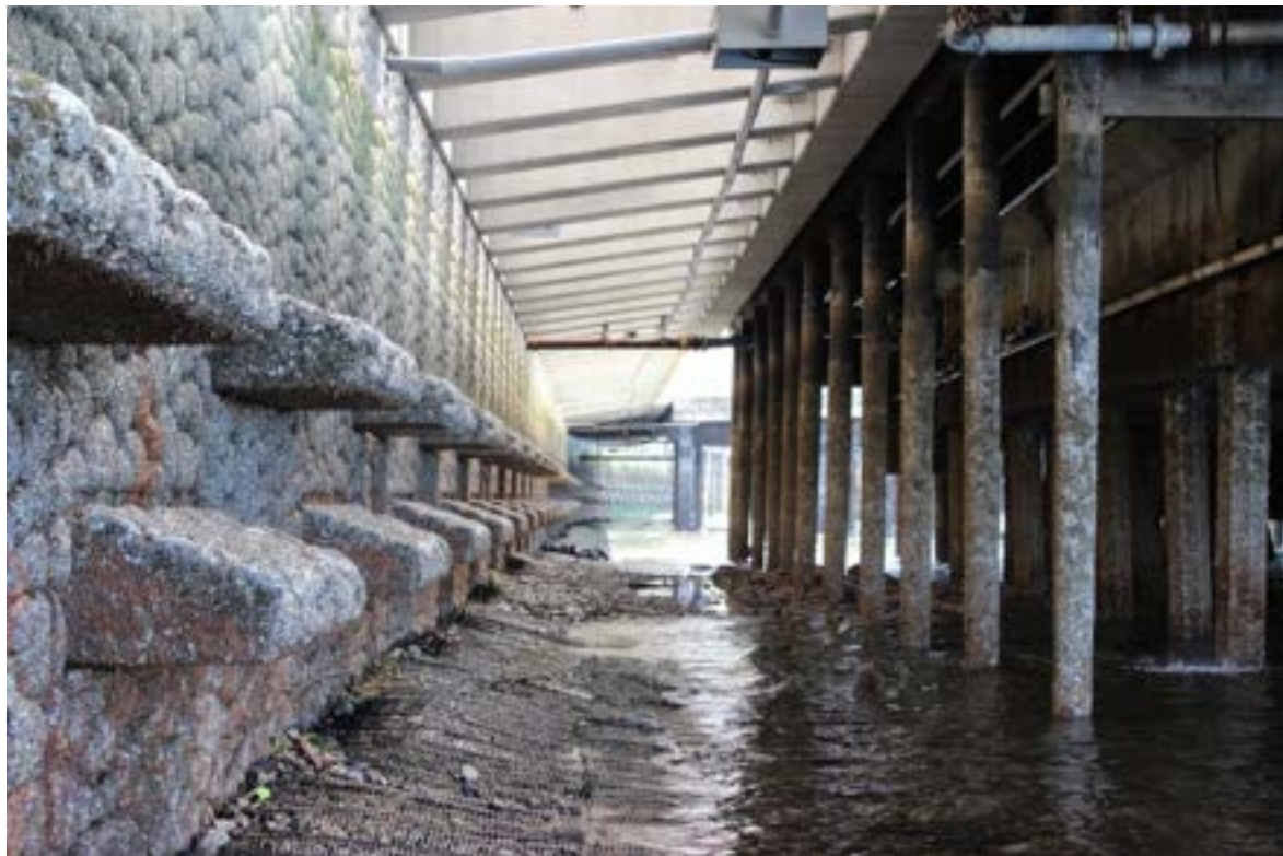
Figure 3. Underneath the Seattle Aquarium pier at low tide, showing habitat enhancements associated with the new seawall—addition of texture and relief to the wall; construction of shallow water benches; and addition of light penetrating glass block surfaces to the sidewalk.
