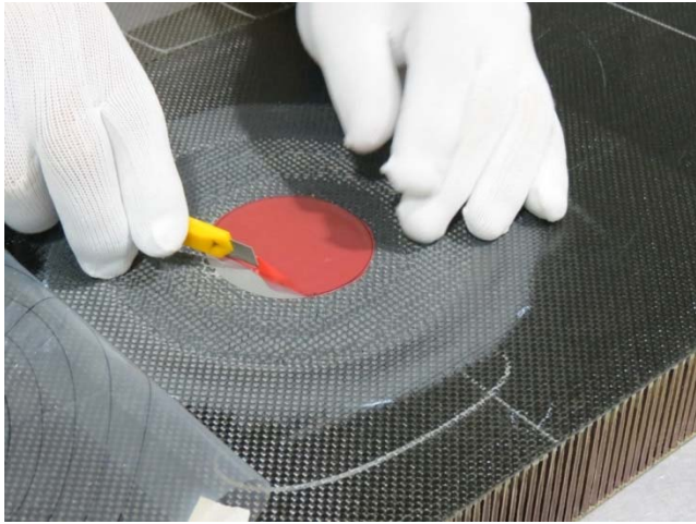
Repair Adhesive Application
