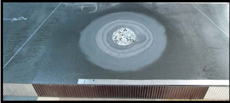
Element scarf sanded in preparation for repair
