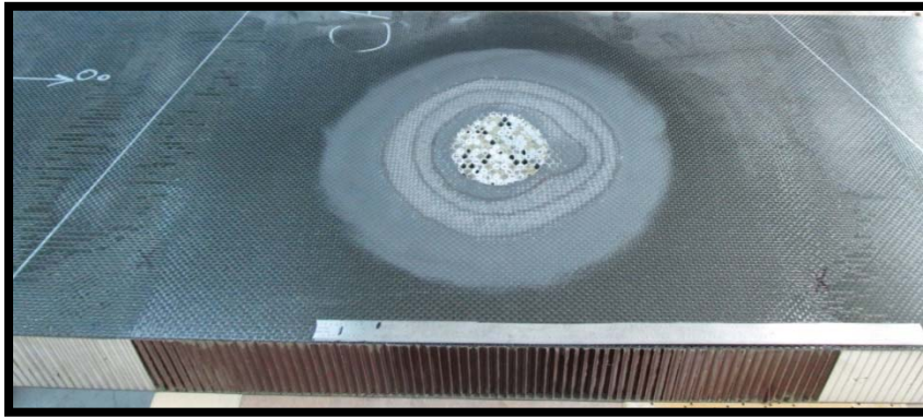
Element scarf sanded in preparation for repair
