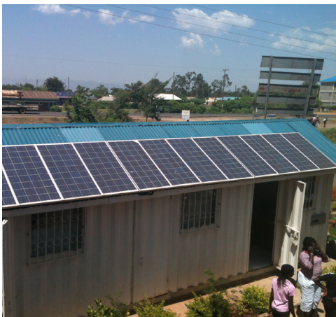
CFAR supported the installation of solar panels to power computer and laboratory equipment in a small research building at the Ahero sub-district hospital in rural Western Kenya, where power outages are common.
