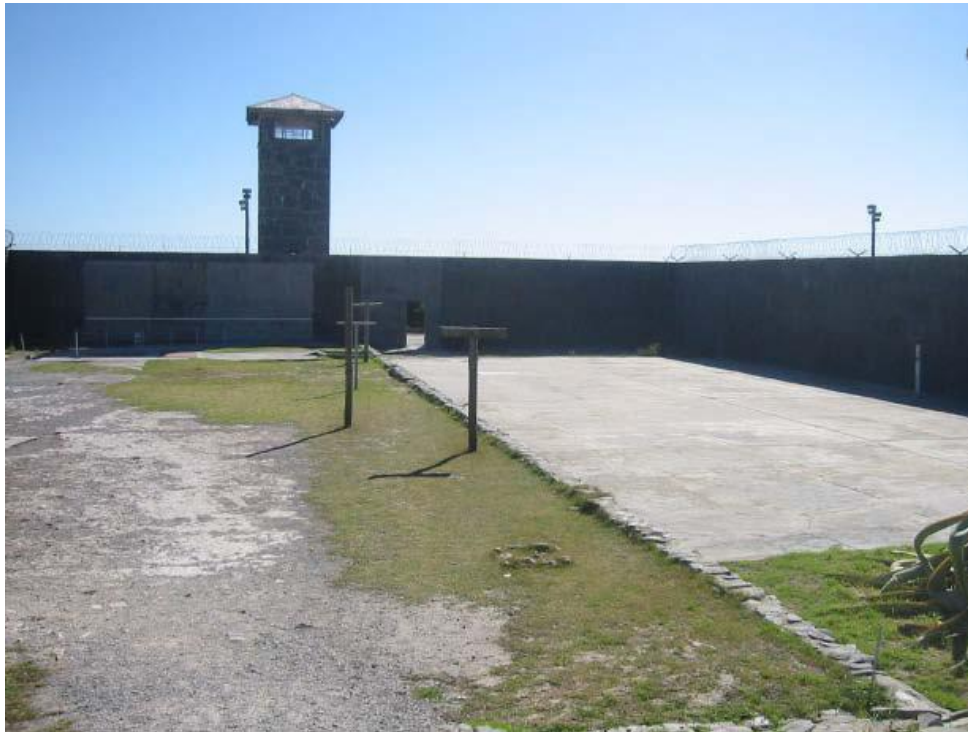
Figure 4. Exercise yard and guard tower at Robben Island
