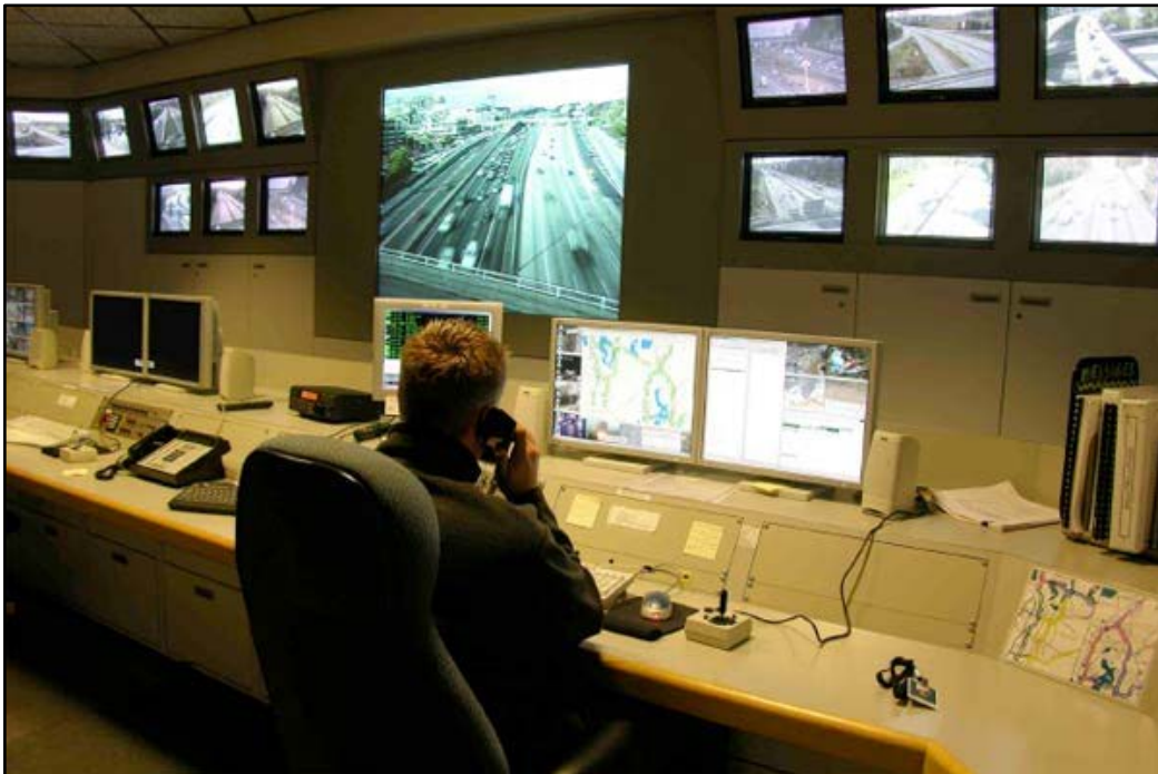
Figure 1: WSDOT Traffic Management Center
