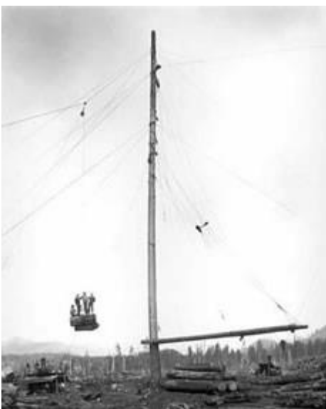
Figure 24: Loading site with donkey engines, spartree, and crew raised in air, Polson Logging Company, near Hoquiam, n.d.
