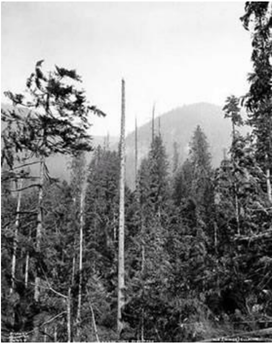
Figure 16: Rigger W. E. Illman on top of topped spar tree, 1929.
