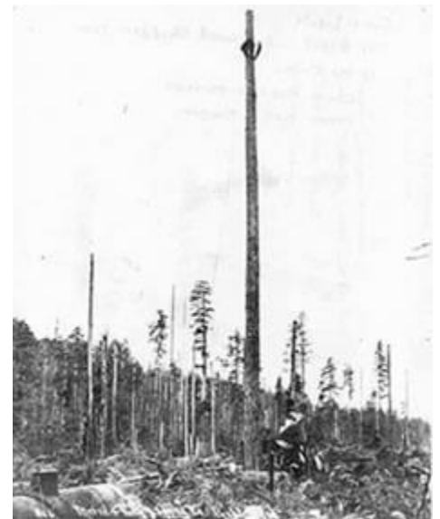
Figure 18 (right): Merrill and Ring Logging Company logging operations where men are rigging a spar tree, probably in Clallam County.
