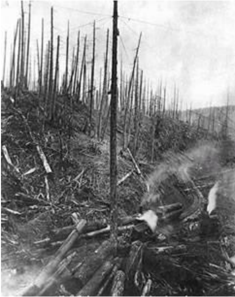
Figure 22: Merrill and Ring Logging Company logging operations showing a spar tree at loading site, probably in Clallam County.
