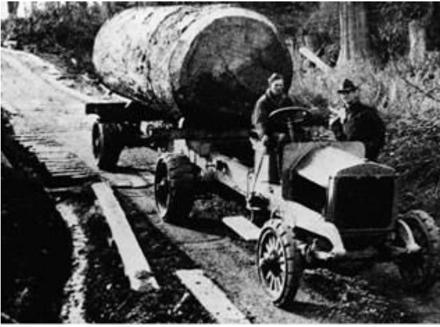
Figure 11 (left) : Diamond-T log truck hauling a large log on a plank road, probably on the
