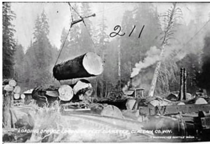
Figure 24: Loading site with donkey engines, spartree, and crew raised in air, Polson Logging Company, near Hoquiam, n.d.
