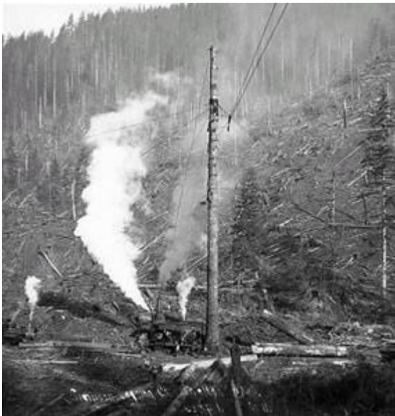
Figure 21 : Loading site with donkey engine, spar tree, locomotive and flatcar, camp 1, Simpson Logging Company, Mason County, ca. 1924.
