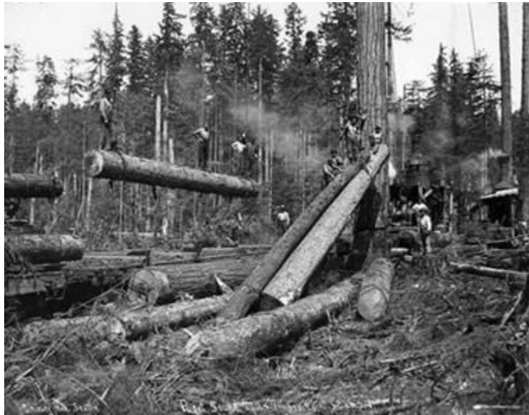
Figure 23: Crew at loading site, with two donkey engines, spartree, and logs suspended above skeleton cars, camp 8, Puget Sound Mill and Timber Company, near Twin, ca. 1922.
