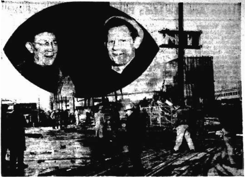
Heroes — Two Portland longshoremen pulled a man from the burning wreckage of the Dock Commission Building the night of November 29 after gas from a leaking 24-inch main blew up the two-story structure. Walter G. Kratt, a construction engineer, was knocked unconscious in the explosion. Local 8 members Lollie Hendricks and J. L. Rucker, left to right in the inset above, were on picket duty nearby at the time. They are credited with saving Kratt's life.
