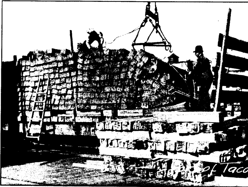
Unloading lath from a flat car with a hammerhead crane at Pier 1, 1925. (Port of Tacoma archives)
