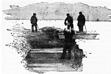
THE TRENCH IN THE POTTER'S FIELD
