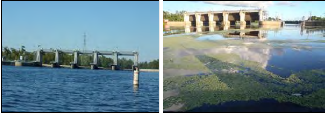
Photo 10. View of the permanent saltwater barrier from upstream (left, November 2011) and downstream (right, July 2012) (photos from Winemiller et al. 2014).
