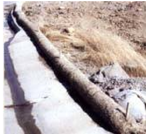
Straw Wattle Installation
