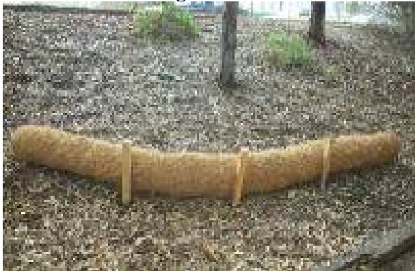
Coir log after Installation
