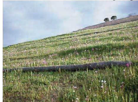
Rice Straw Wattle on long slope
