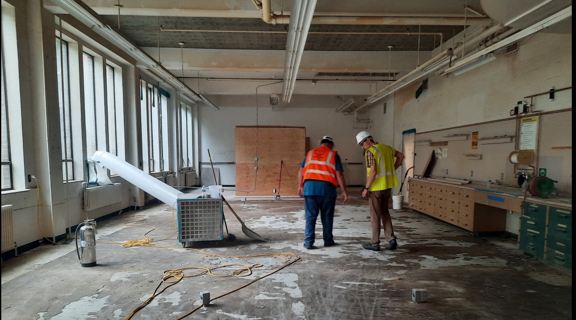
Former Woodshop space after demolition
