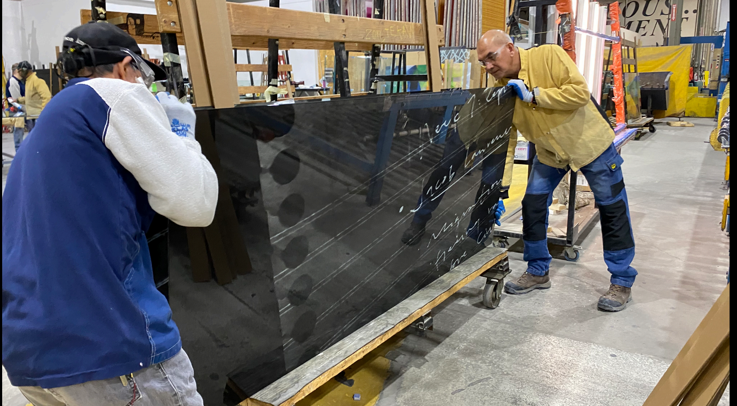
Fritted glass for the new Jacob Lawrence Gallery windows
