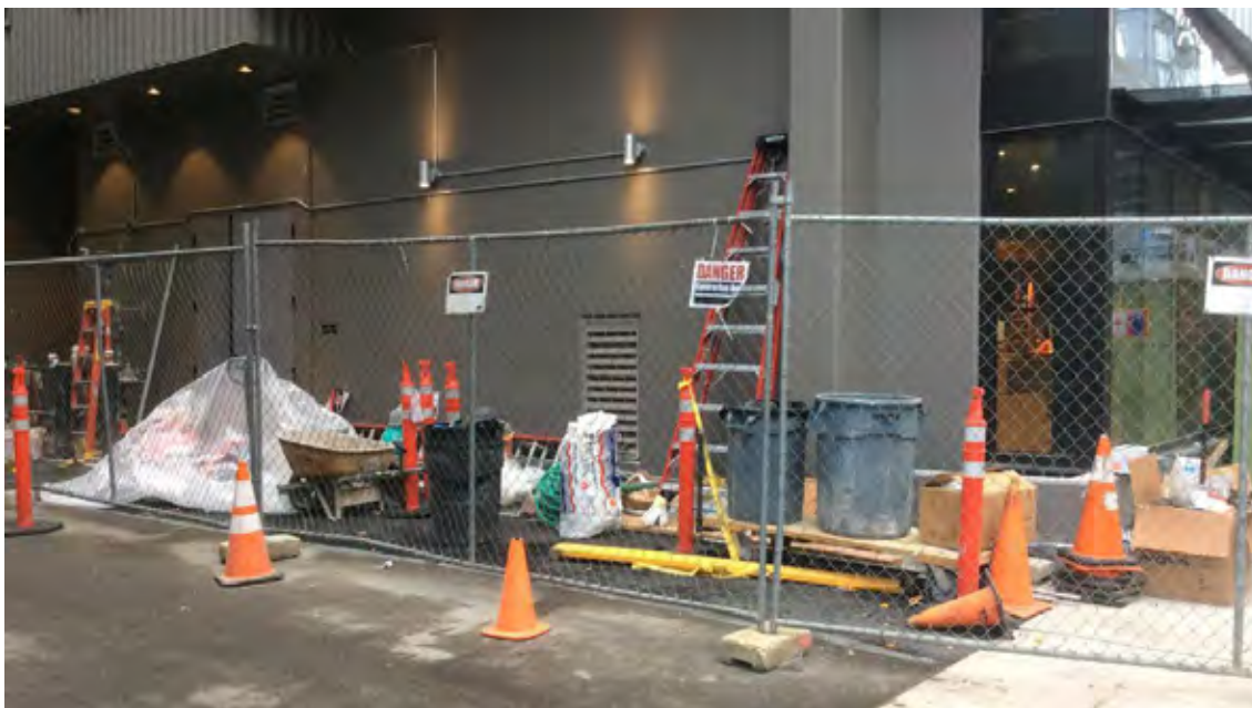
Figure 1-13. An Alley Blocked by Construction
