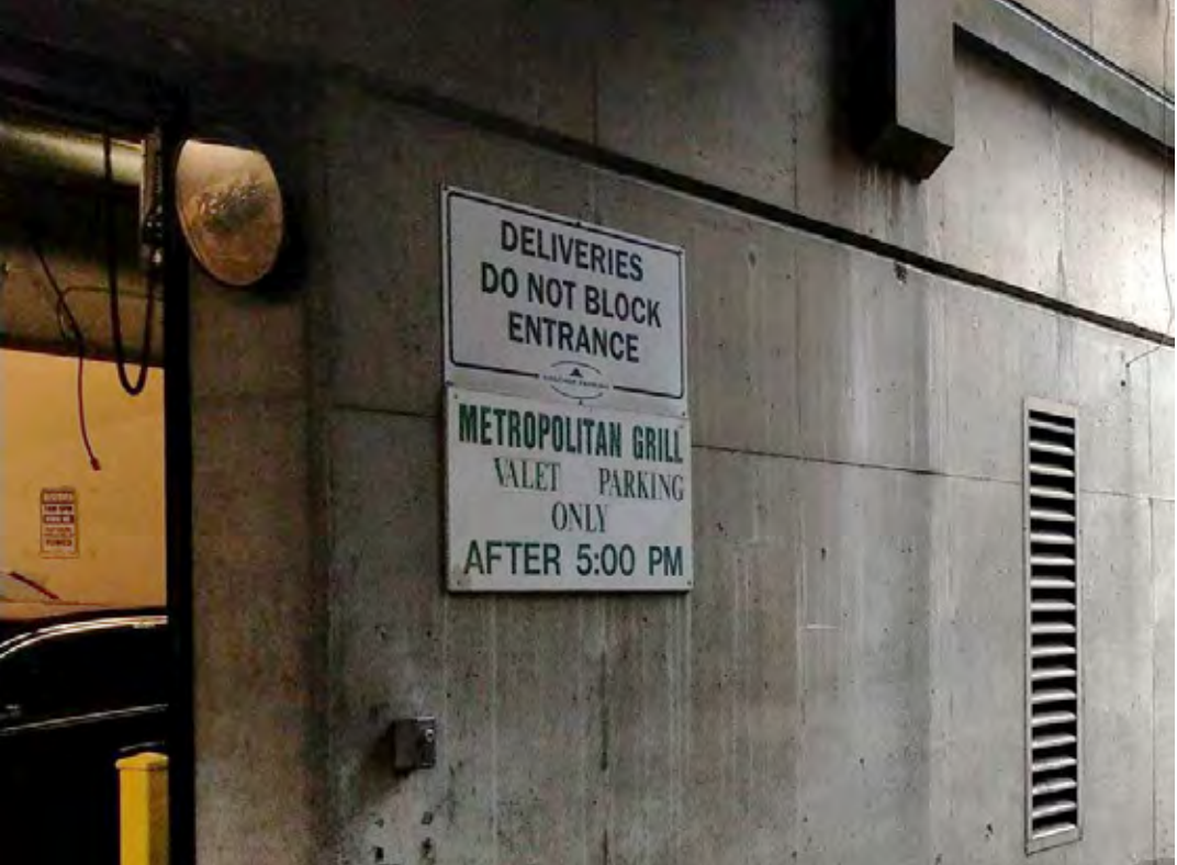
Figure 2-22. Signage Inside the Alley
