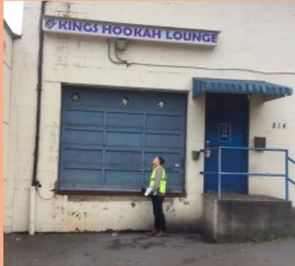
EXTERIOR LOADING DOCK
