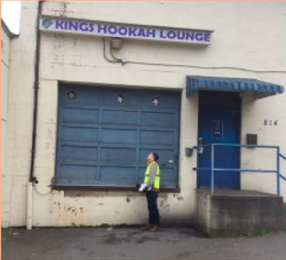
EXTERIOR LOADING DOCK
