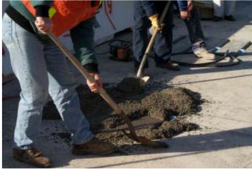
Figure 4.3. Placing Grout in Dowel Bar Slots (Image Courtesy Pavement Interactive)
