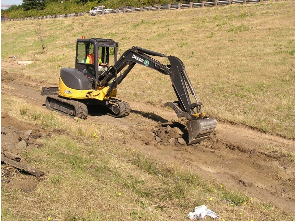
Figure 24. Excavator removing asphalt lining in ditch
