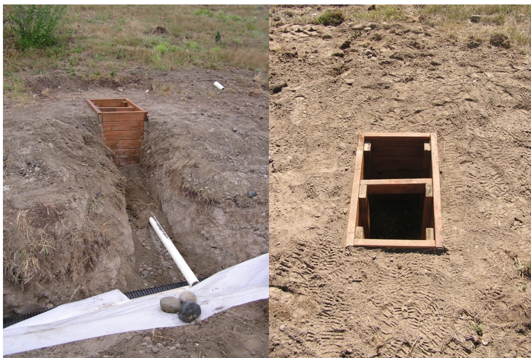
Figure 25. Wood box for TB3 pit rain gauge showing drain to French drain (left) and fully installed
