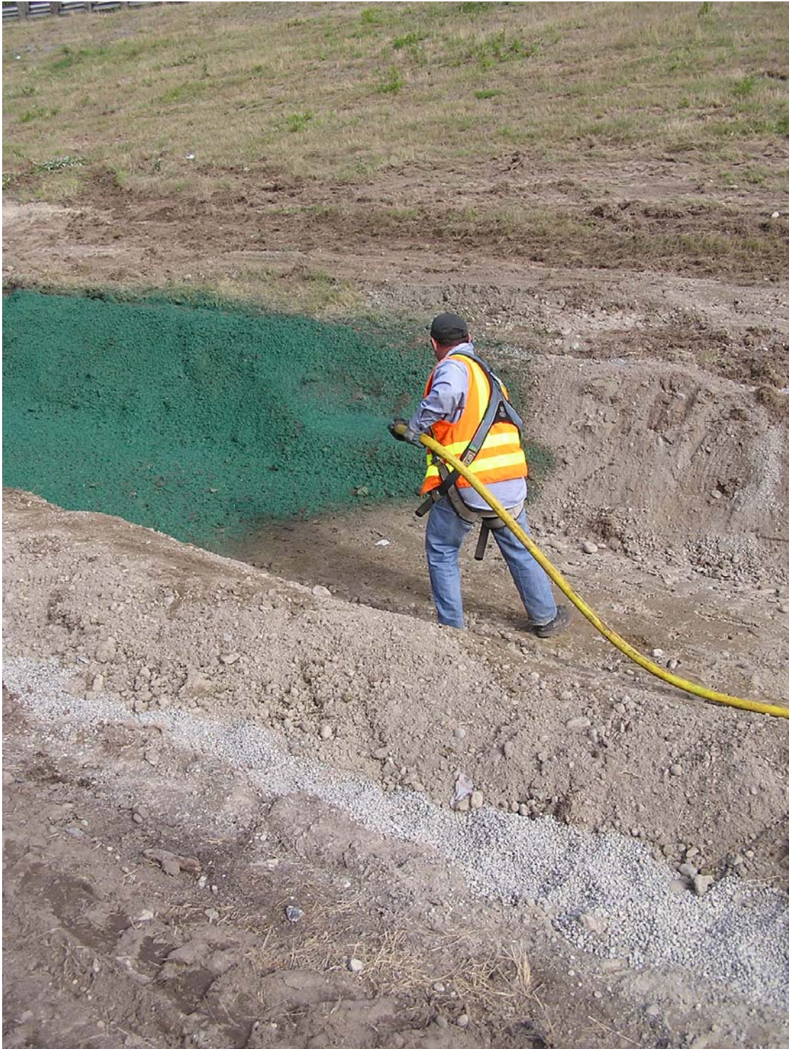
Figure 31. Hydroseeding Bioswale 2 with hose
