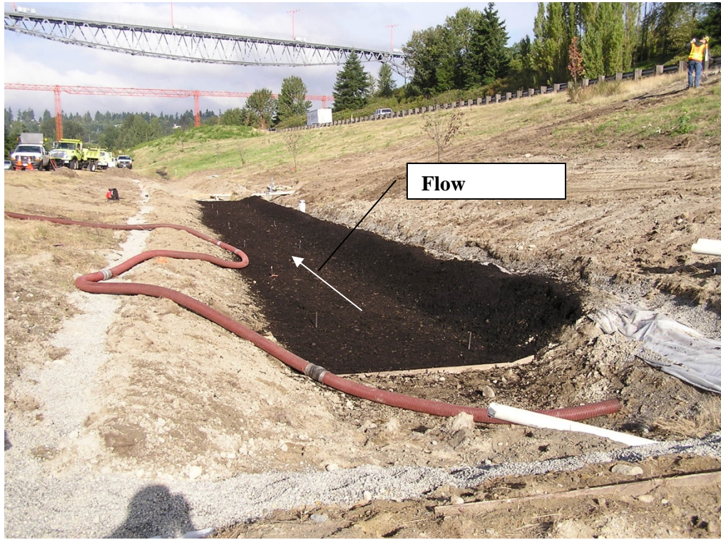
Figure 29. Bioswale with compost blanket installed
