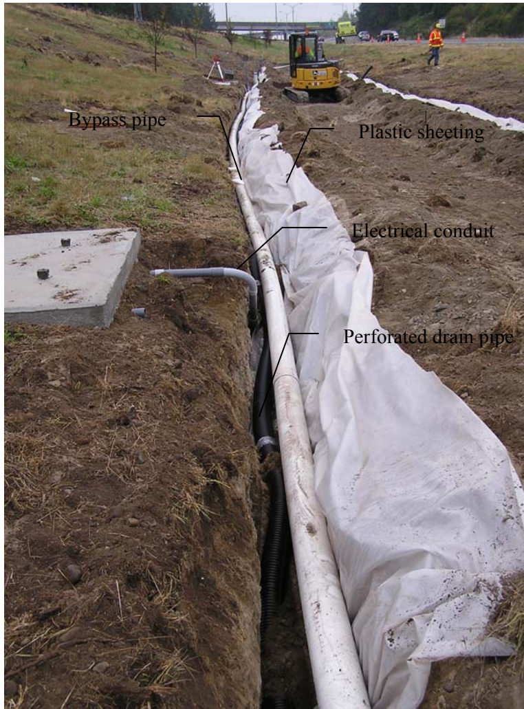
Figure 13. French drain trench with plastic sheet lining, perforated (black) and solid pipe (light), and electrical conduit installed
