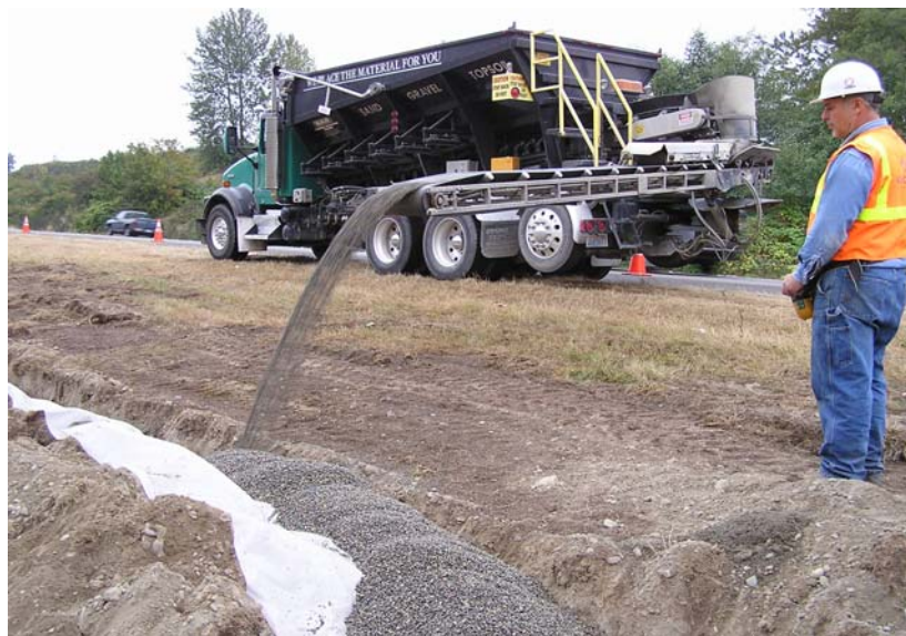
Figure 17. Pea gravel being placed in French drain by an aggregate delivery truck
