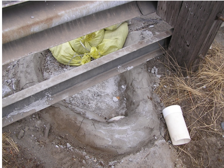
Figure 16. Curb cut and inlet pipe with temporary cap removed and flow blocking sandbags in place
