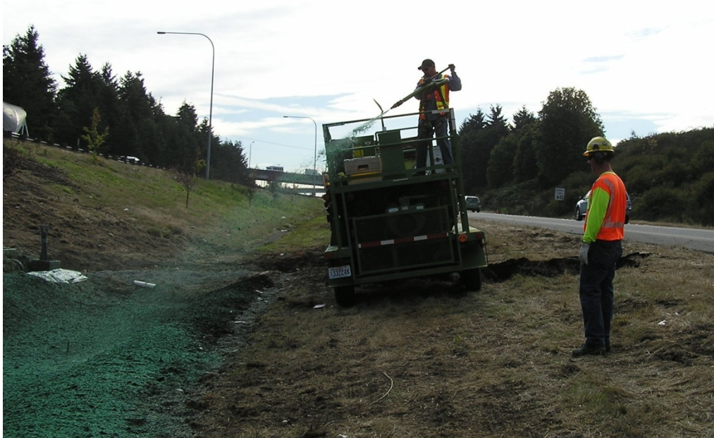
Figure 30. Hydroseeding Bioswale 1 with trailer mounted nozzle
