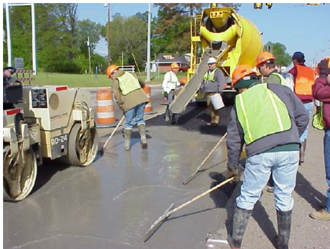
Figure 18: Excess grout worked into areas needing more (Battey and Whittington 2007).
