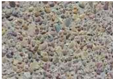
Figure 19: An exposed aggregate surface (Silent Roads, 2003)
