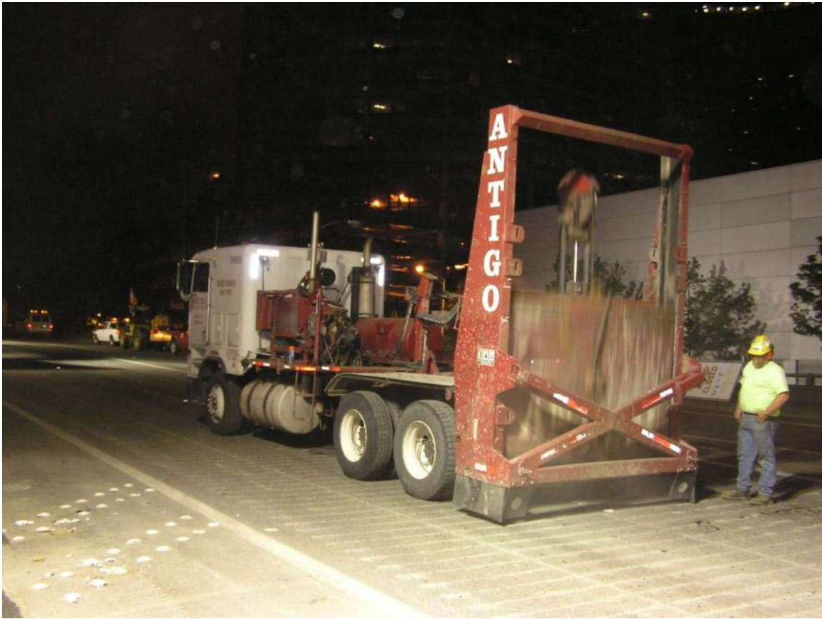
Figure 11. Drop hammer truck.
