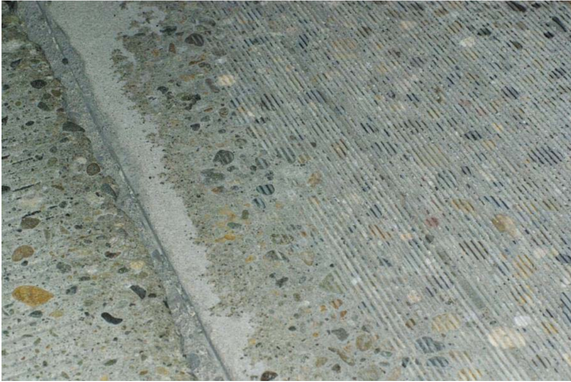
Figure 8. Pavement surface after diamond grinding (right side).
