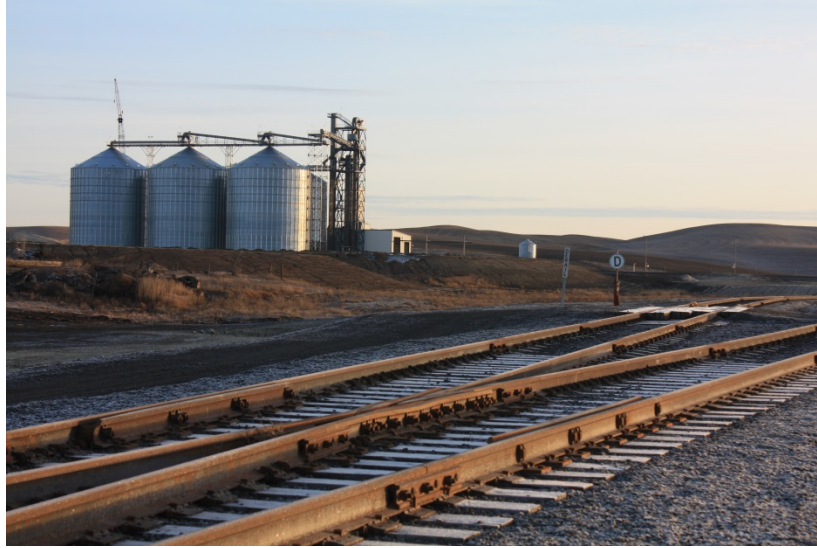
Figure 6. McCoy Grain Loading Facility.
