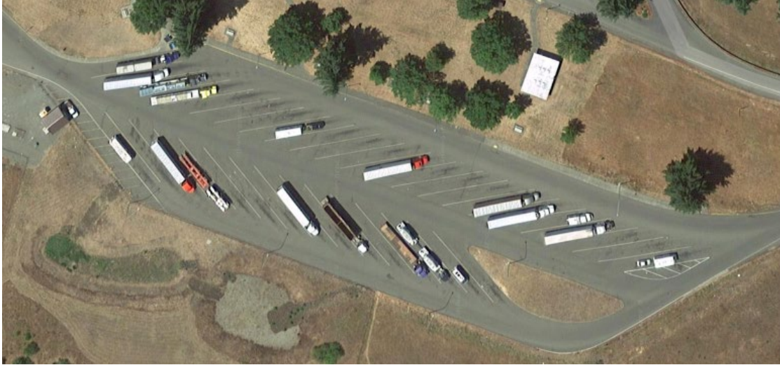
Figure 4–3. Scatter Creek Safety Rest Area Truck Parking Lot Overview
