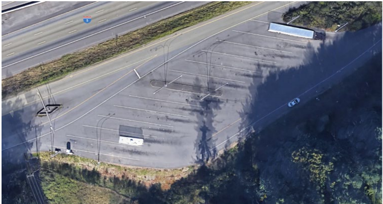
Figure 4–2. Nisqually Weigh Station Truck Parking Lot Overview
