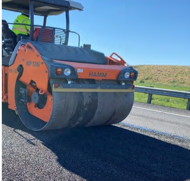
Figure 3-6. Photo. Oscillatory Roller.
