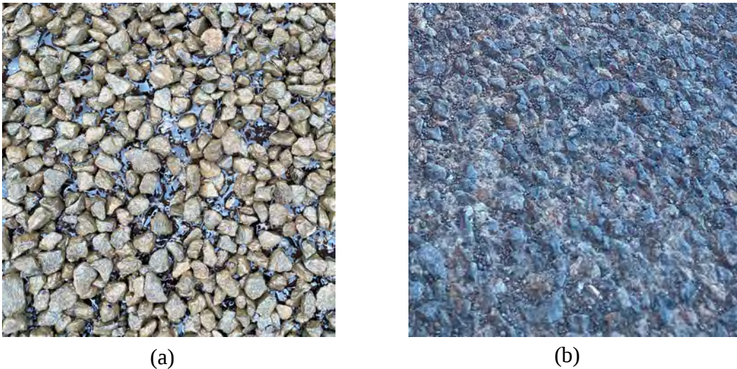
Figure 4-38. Photo. Surface Texture of SR 142 without Choke: (a) During Construction; and (b) After One Year.
