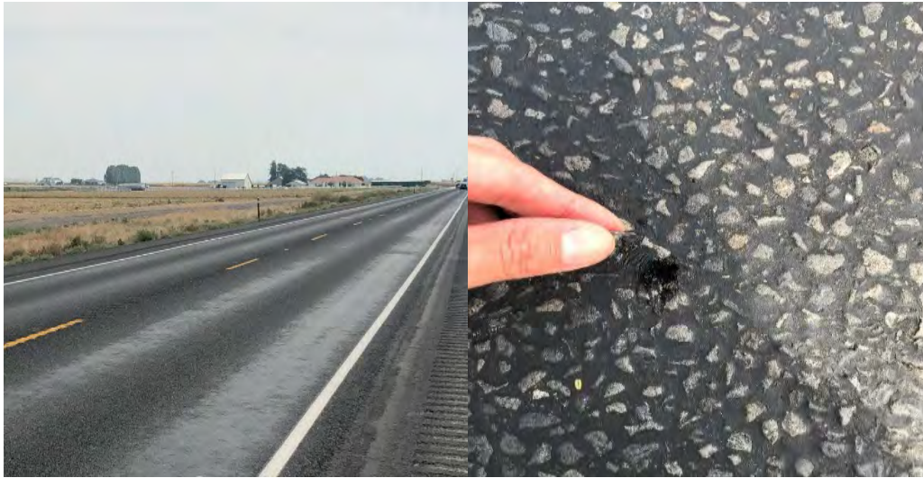
Figure 4-25. Photo. SR 17: (a) Bleeding in the Wheelpath and (b) Close-up View.
