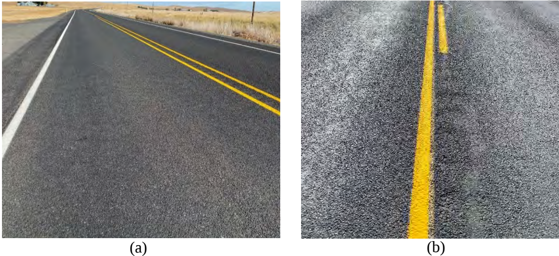
Figure 4-9. Photo. Condition on SR 127: (a) Chip Seal Over New HMA; and (b) Chip Seal Over Existing Chip Seal.
