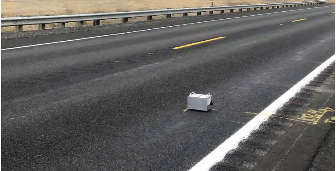
Figure 4-6. Photo. Bleeding in the SR 26 Wheelpath.
