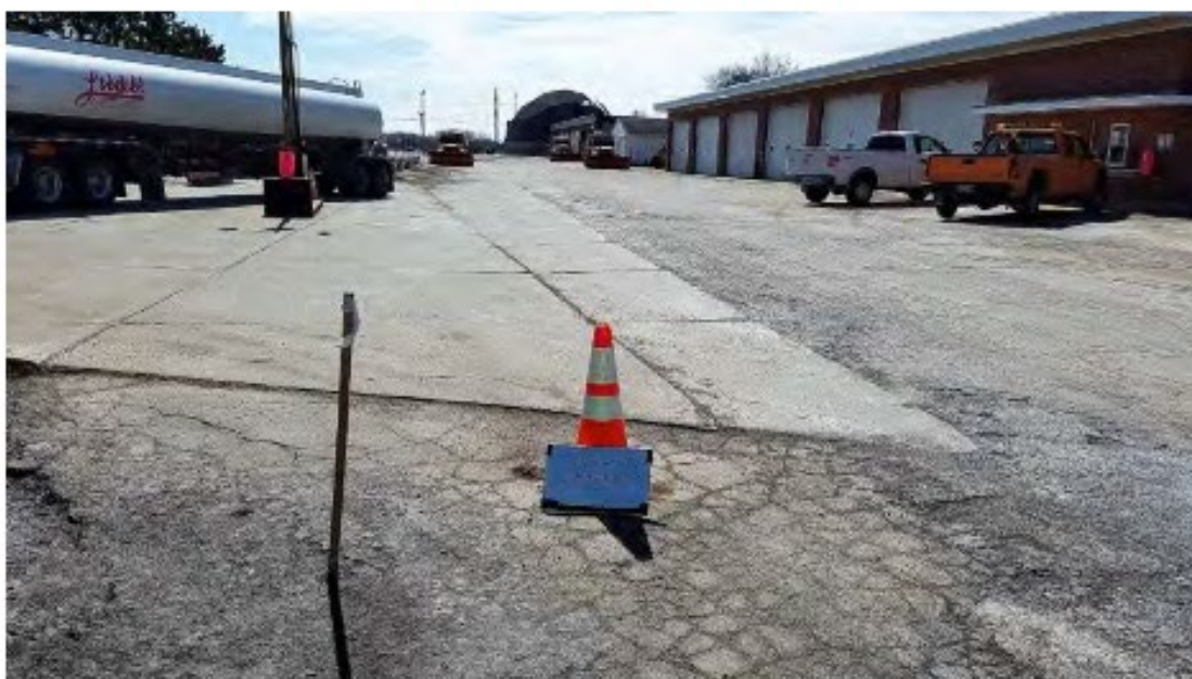
(B) Boring 244-B14, facing south
